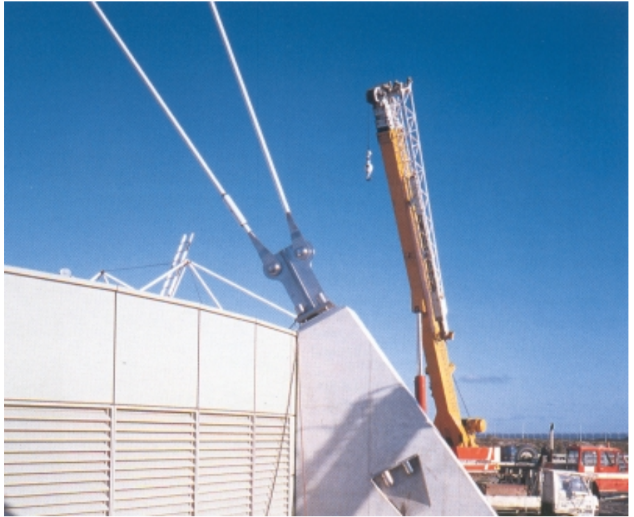
Above: Tower guys connecting to concrete buttress through clevis plate.
