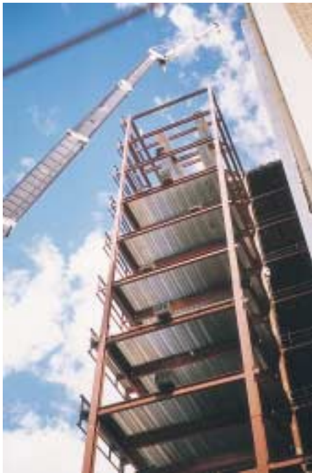
Structural steel frame under construction.
