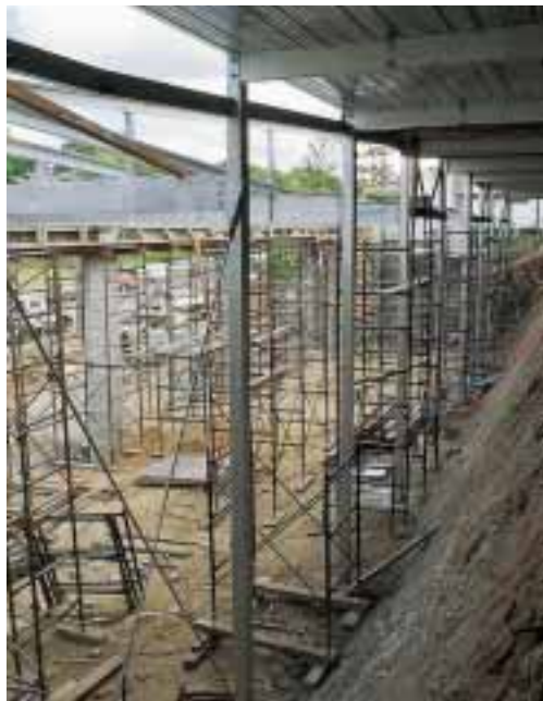
Left: Bondek flooring supported on steel beams
