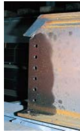
Figure 11. New stringer, showing new end design to prevent fatigue cracking.
