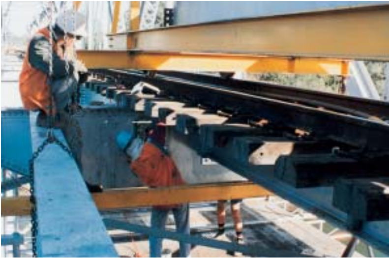
Figures 9 and 10. Removal of old, and installation of new beams at Boyne River bridge, showing underslung scaffold for safe working access.
