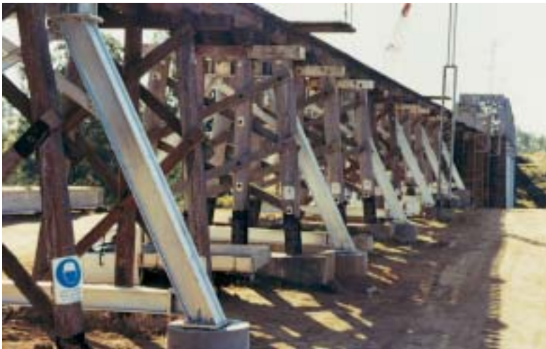
Below: Figures 2,3,4. Mary River bridge, showing erection of substructure steel, and changeover erection of new steel spans.
