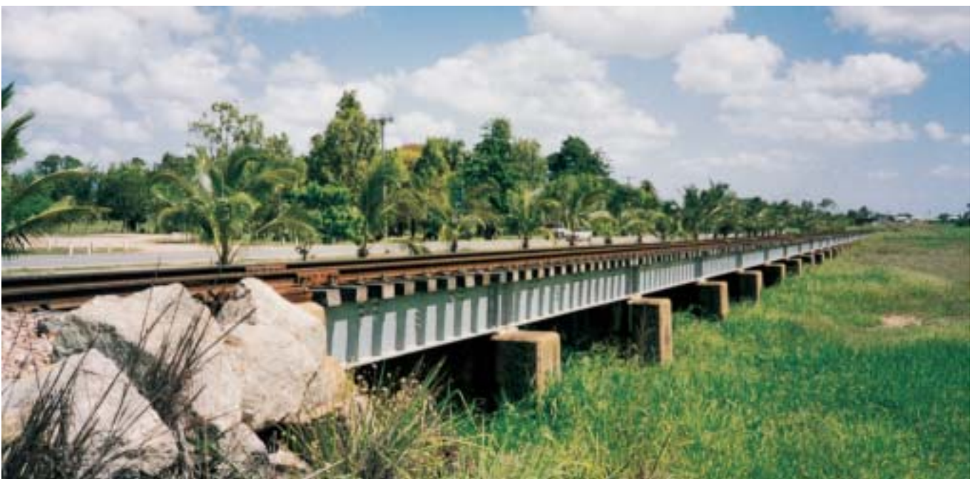
Figure 14. Plantation Creek bridge.
