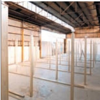
To allow ease of assembly and to assist levelling on the uneven slab, the DuraGal bearers were supported over the columns using standard adjustable top fittings from the DuraGal Flooring System.
