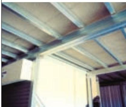
to form a skillion just above the mezzanine floor. The portal rafters were joined to the columns with knee bracing as shown in the following photograph.
