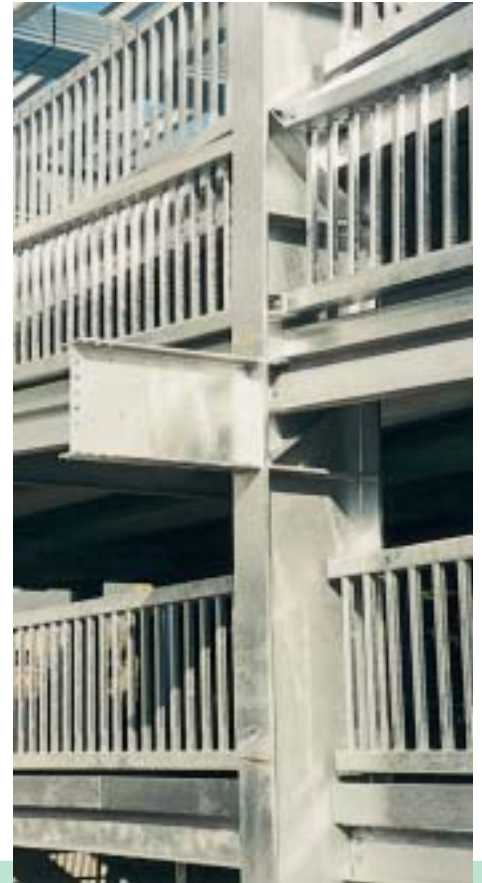
Columns prepared with beam 'stubs' provide large spans, improving footing costs and ease of parking.
