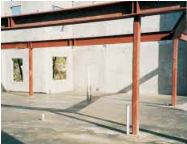
Steel construction combined with external concrete tilt-up panels.
