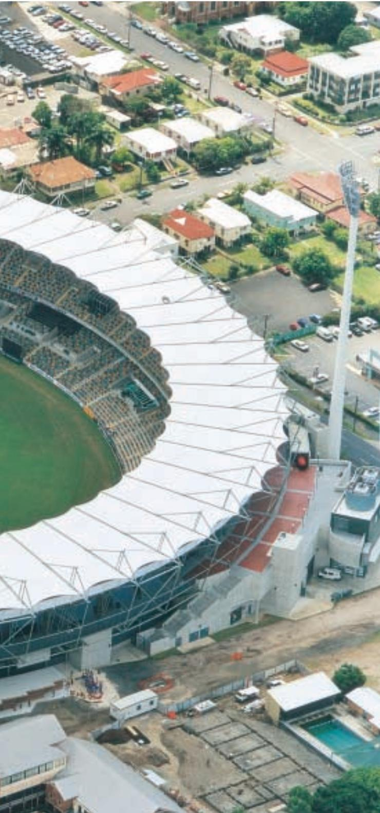
The raking girders and steel beams are supported on steel columns comprising circular hollow sections and universal columns. Precast pre-tensioned concrete seating plats span distances of 8m to 11m between the raking steel girders. The horizontal floors (Levels 3 and 4) beneath the seating tiers comprise 250mm and 300mm thick precast concrete hollow-core panels, also spanning 8 to 11m, and topped with 75mm thick concrete.
