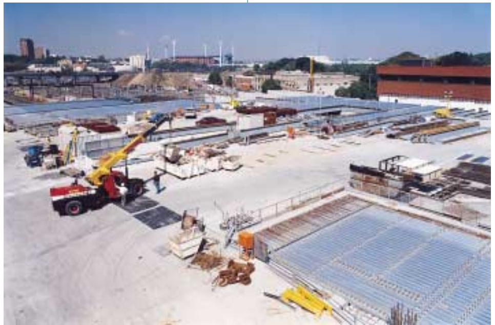
Above: Beams stacked on concrete deck for next erection session.
