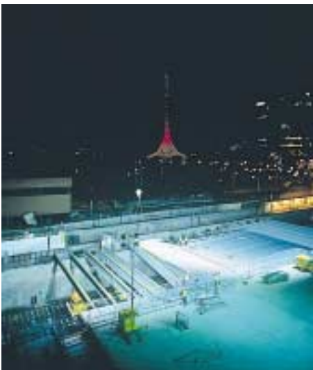
Welded beams being placed during night occupation.
