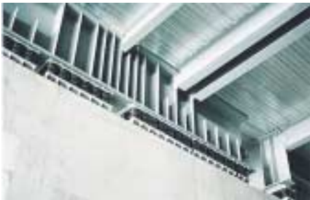
View from under deck showing isolating bearings.
