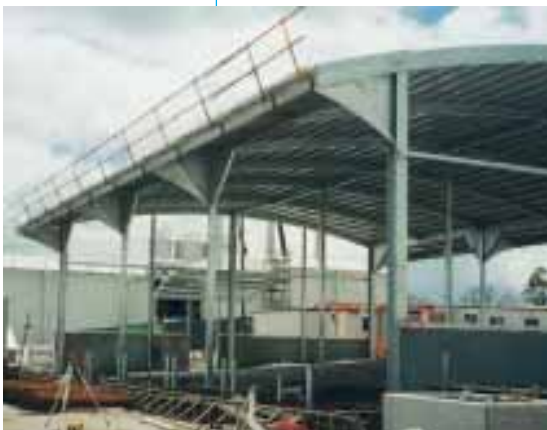
Bonlac's new processing plant under construction
