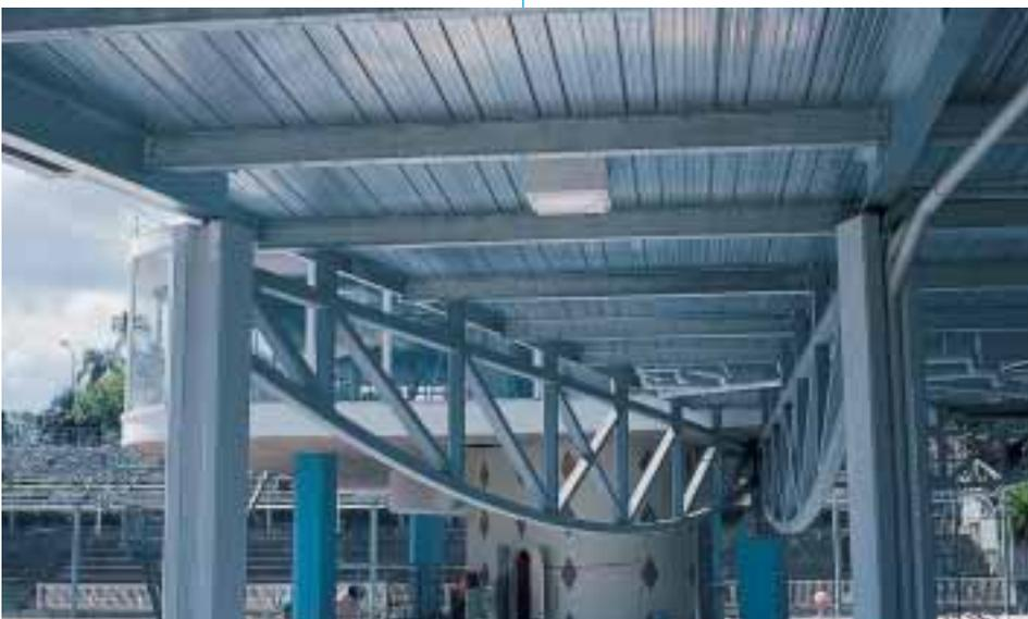
*Bowstring truss and Bondek composite flooring at the Centenary Pool redevelopment.*
