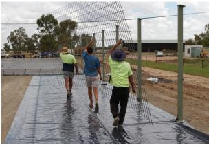
To accommodate the expansion plans of Australian poultry giant Baiada, Yoogali Concrete Constructions has completed the first two of four chicken shed concrete slabs using a special size mesh from OneSteel Reinforcing.
